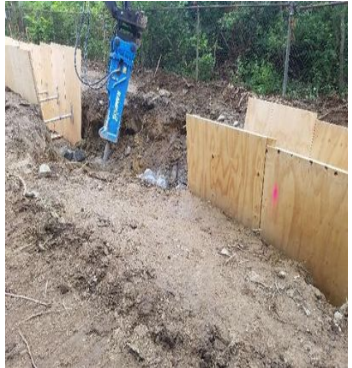
Fig 6: McCourt continues to hammer ledge next to field house. Viewing northeast. (6-27-19)
