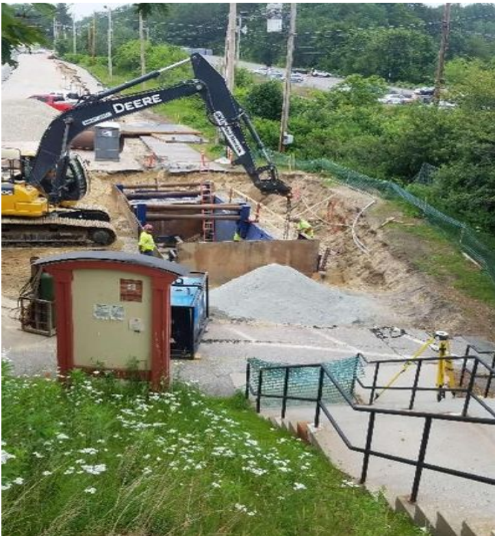
Fig 7: Midwest Mole Inc. continues to drill in jacking pit. Viewing north. (6-27-19).
