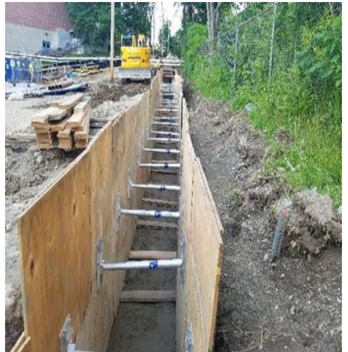
Fig 16: Trench next to Colovos Rd, heading towards steam pipe. Viewing north. (7-01-19).
