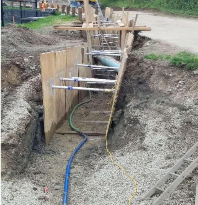
Fig 1: McCourt continues to trench along Colovos Rd, moving north. Viewing north. (6-27-19).
