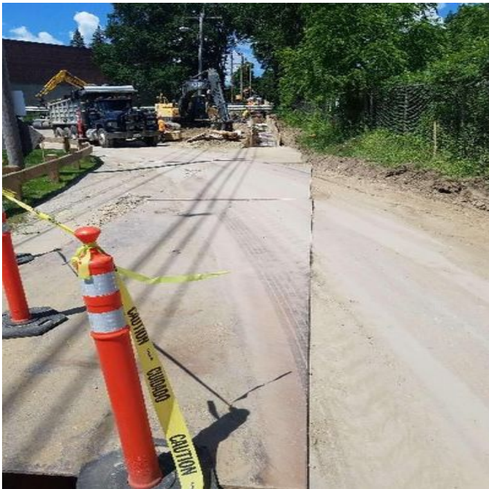
Fig 11: McCourt continues to excavate along and across Colovos Rd. Viewing north. (6-28-19).
