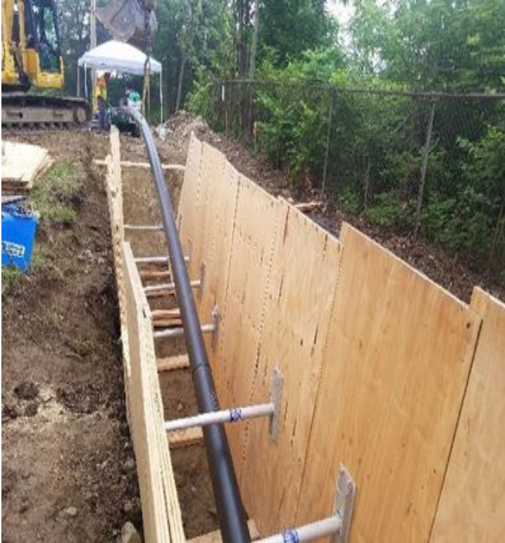
Fig 9: McCourt fusing pipe in trench next to field house. Viewing north. (6-28-19).
