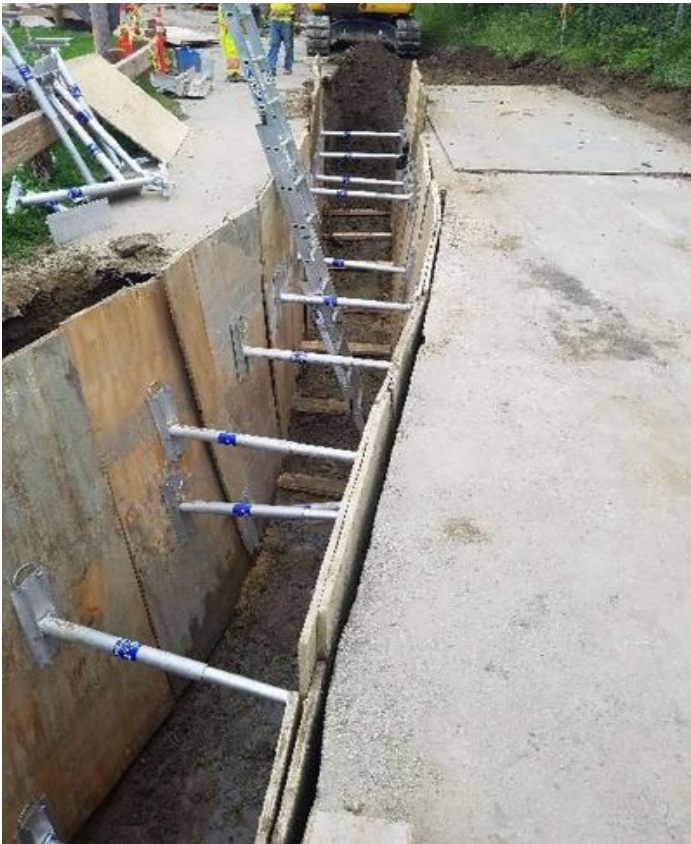
Fig 3: Trenching across Colovos Rd. Viewing north. (6-27-19)
